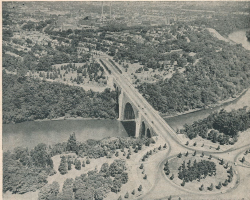
Air View of Rochester Memorial Bridge
